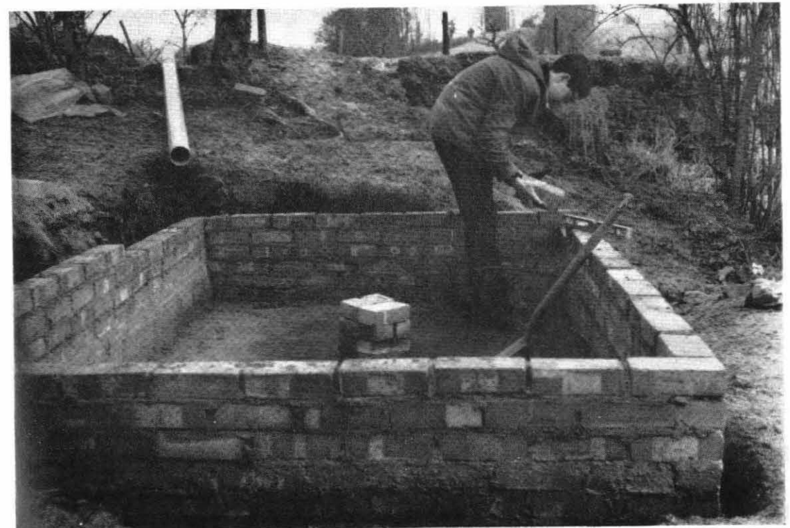
THE TROUT HATCHERY Two Stages during the laying of the foundations
